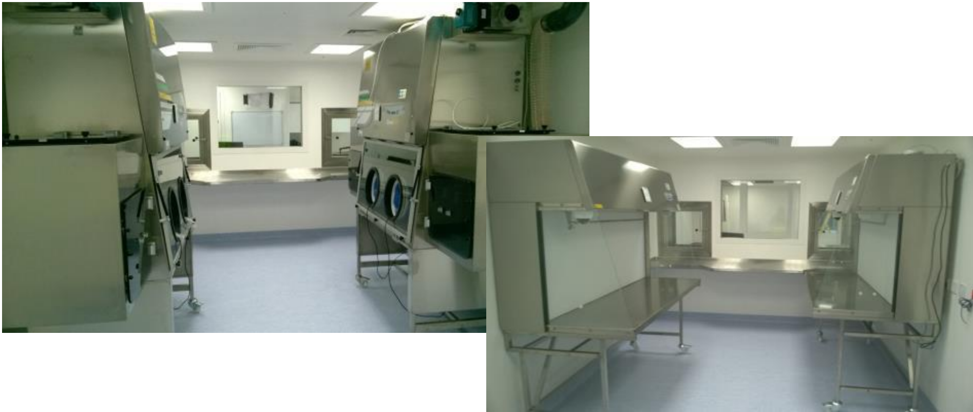
Cytotoxic isolators and LAF cabinets fully made in stainless steel, Ulster Hospital - Northern Ireland
