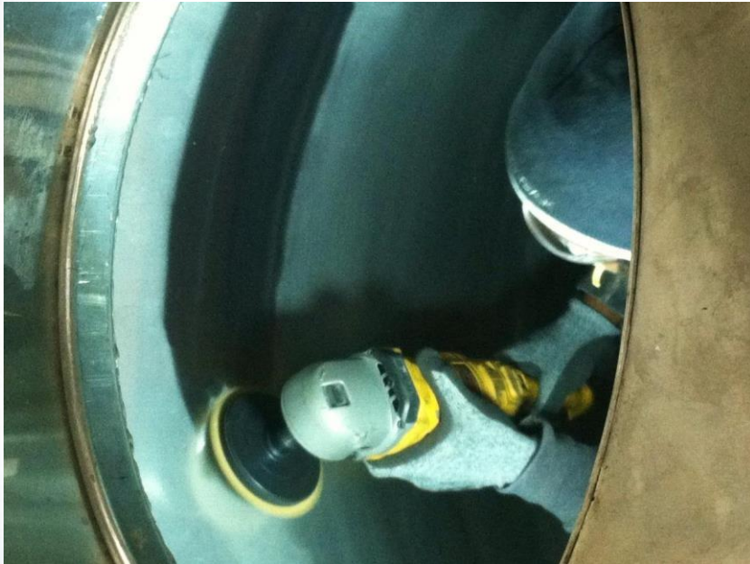
MP technique performed in-situ in vessel
